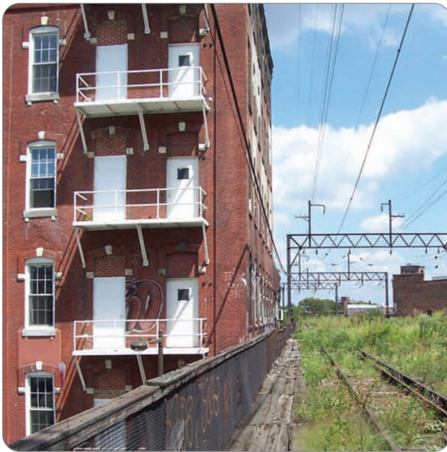
Northeast view at Ridge Avenue and Noble Street. Built in the 1890's the viaduct is a combination of embankment sections, bridged by steel structures and arched masonry bridges.
